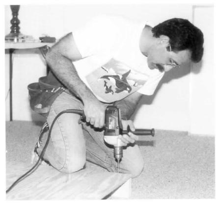
Use a drill with a Phillipshead attachment to turn the screws into place. The end screws should be an inch or so from the ends, and the rest should be about 8 inches apart.
