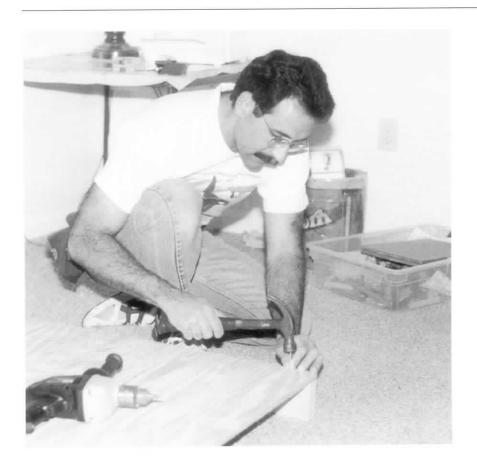
Use 3-inch deck screws to secure the plywood to the frame. Start the deck screws by hammering them slightly into place.
