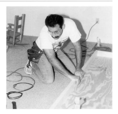
To complete the frame, flip the train board over again and add three additional interior lengths. Be sure to mark the locations of these interior frame members on the ends of the outer frame so that you can transfer the marked locations to the plywood surface. Since the control board length is 45 inches, the distance between the outer faces of the two end frame members needs to be this distance.
