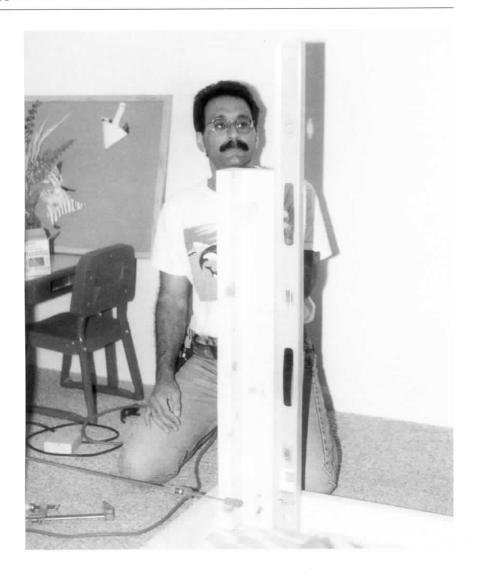
At this point angle braces, cut at 45-degree angles at both ends, have been added. This end is now done, and pretty soon it will be time to add the control board. Note that in order for the 45-degree braces to sit flush against the frame you have to add an additional length of wood to the back side of the frame.
