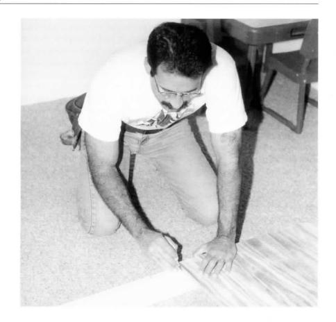
After cutting (wearing safety glasses, of course) the 2 x 4s to your marked lengths, position the cut 2 x 4s under the 4-foot ends of the plywood and mark the locations for the screws.
