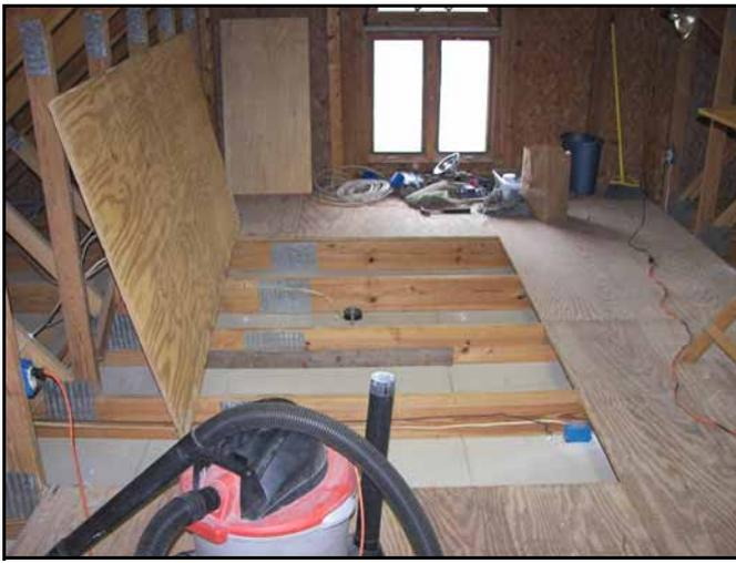
The first construction step after clearing out the area was to pull up the existing 3/4 inch plywood flooring so that I could add R-19 insulation. My hands were a bit sore after pulling out all those nails!
