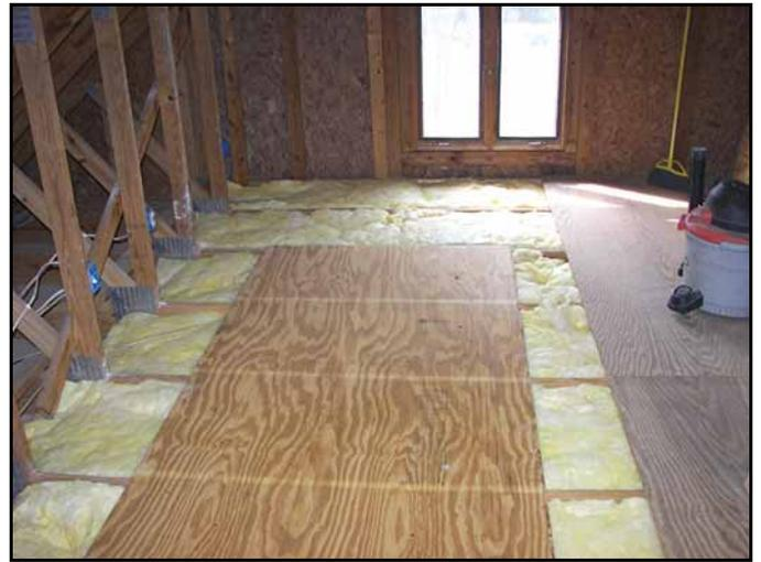
The floor insulation was installed face down and I stapled the edges along the sides of the floor joists. I then carefully nailed the floor sheathing back down.
