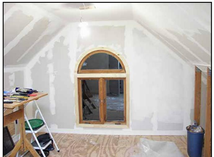
I added fiberglass mesh tape to the seams and corners and then gave them 2 coats of mud. I added the trim work and then I diluted the mud a bit so that it would flow better and I applied it to the entire surface of the ceiling and the walls.
