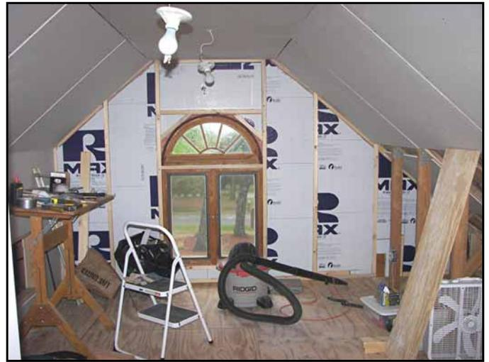
The existing window wall was insulated with several layers of 3/4 inch foam insulation. Once the insulation phase was complete I started adding the wallboard to the ceiling and then the walls.
