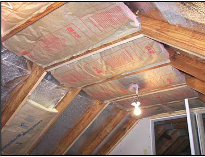
Once all the framing was completed it was time to insulate the ceiling and the walls. I used R-30 for the ceiling and R-11 for the walls.
