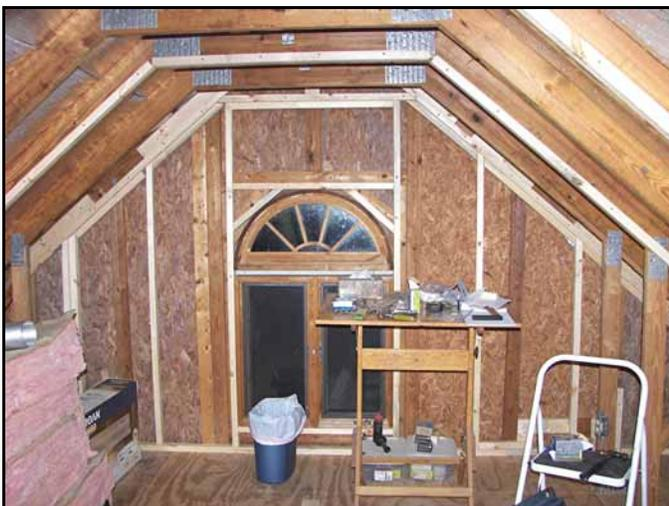
Next I framed out the window wall so that I could add foam sheet insulation and then the wallboard. I also added extra nailing lips to every other truss so that each wallboard seam would have a 3 inch nailing lip.
