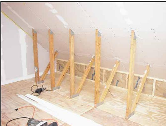
It took some time to carefully measure and cut each section of wallboard and then form fit each piece into place to get a tight fit. Adding wall mud to all the seams was a real challenge.
