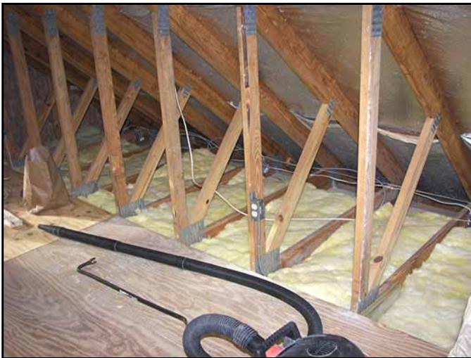
I wanted to expand the flooring to one side of the truss work so that I could use it for storing my unbuilt model collection. Here the insulation has been added and the wiring has been moved to the extreme end of the floor joists.
