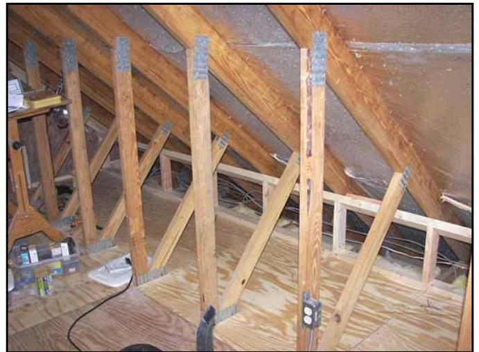
I carefully cut sections of 3/4 inch plywood and form fitted them into place around the truss work. I also built the small wall which I had to construct twice before I got it straight and level because the trusses were slightly off center.
